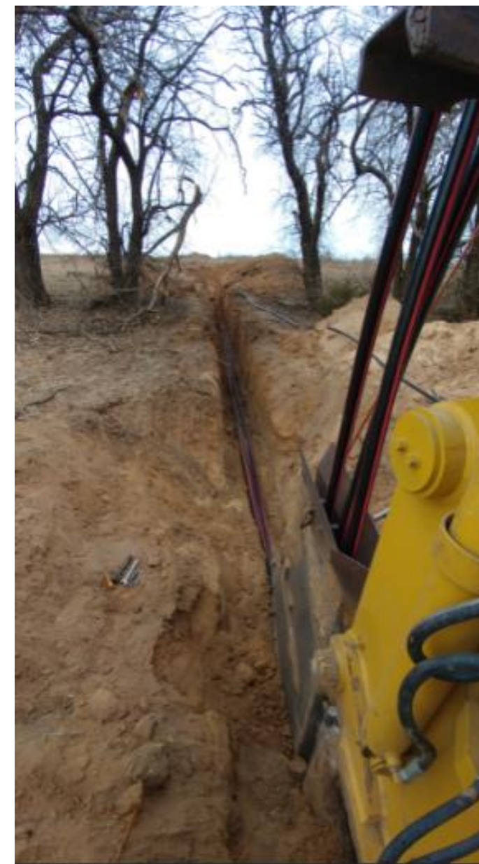
34.5- kV underground trench, approximately 42" deep. Slide 21
